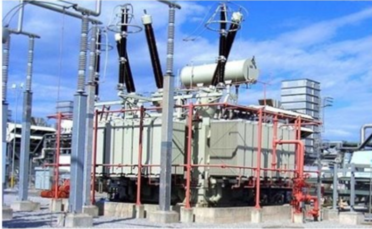
Figure (1) Medium power transformers (cgglobal, 2016)
